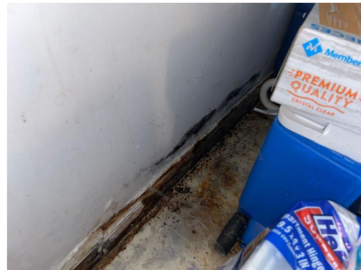
Interior Kitchen South lower drywall, wood baseboard Visible water damage Visible microbial growth (>10 sq ft)
