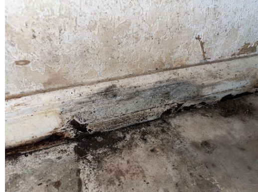
Interior Garage West lower drywall, wood baseboard Visible water damage Visible microbial growth (>10 sq ft)
