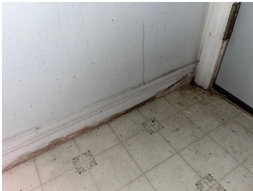
Interior Kitchen East lower drywall, wood baseboard Visible water damage Visible microbial growth (>10 sq ft)
